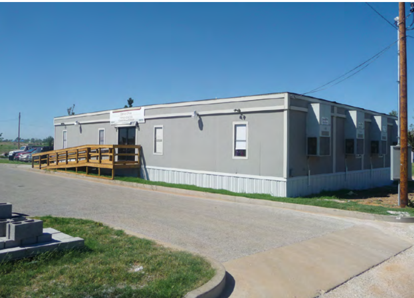
Four trailers served as temporary space while the new office was designed and built
